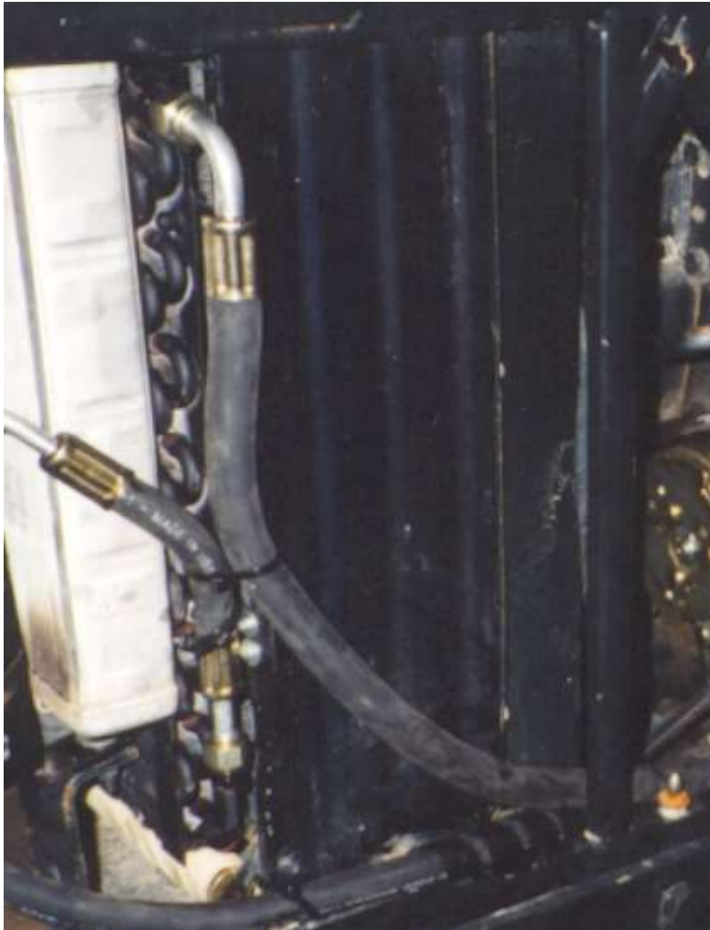
Condenser in place with hoses shown.
