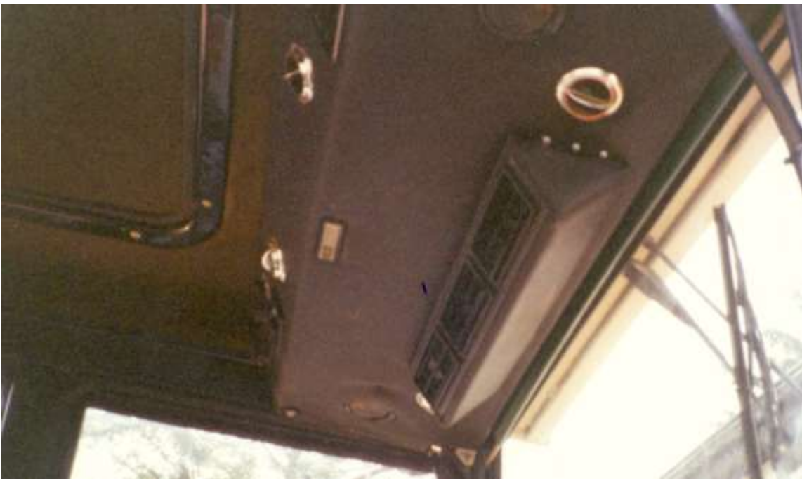
Air distribution panel also showing the recirculation louvers (chrome louvers no longer used – just factory louvers originally in place).
