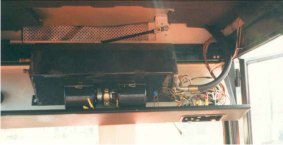
Heat/cool box in position with blowers remounted.
